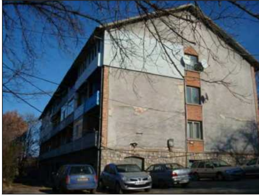
Exterior view of the building
