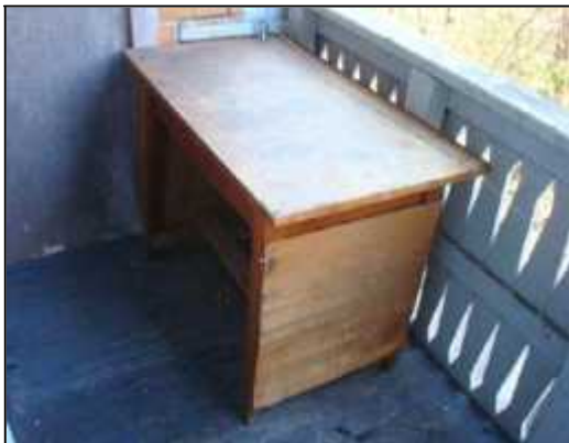
Interior view of the balcony
