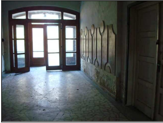
Interior view of the entrance
