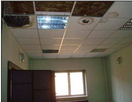
Interior view of the suspended ceiling
